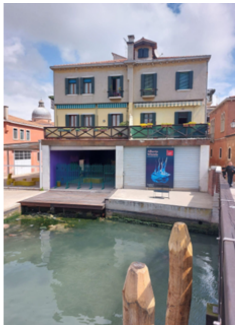
Figure #1: deep dive (pause): uncoiling memory at the Docks Cantieri Cucchini. Image taken on 26 April 2022 by author.
